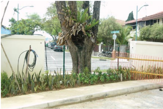
Boundary fencing was offset 300mm to preserve the tree
