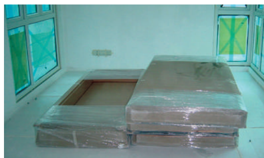
Figure 5.4 Door panels and frames should be sent directly to the units where they are to be installed
