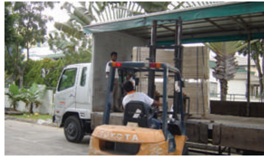
Figure 5.2 Materials transported in covered vehicle and under good weather conditions
