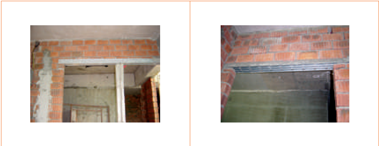
Figure 2.1 Types of lintel used for door opening
