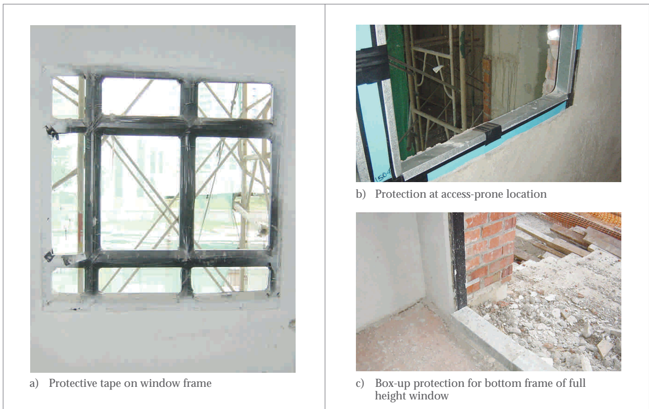
Figure 8.2: Protection of frame throughout construction process
