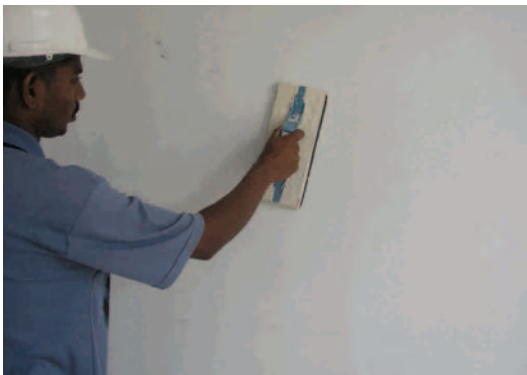
Figure 5.1 Sanding between coats of paints
