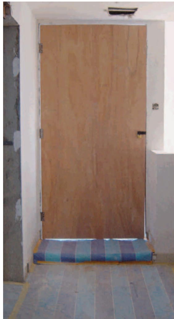
Completed work protected by restricting access
