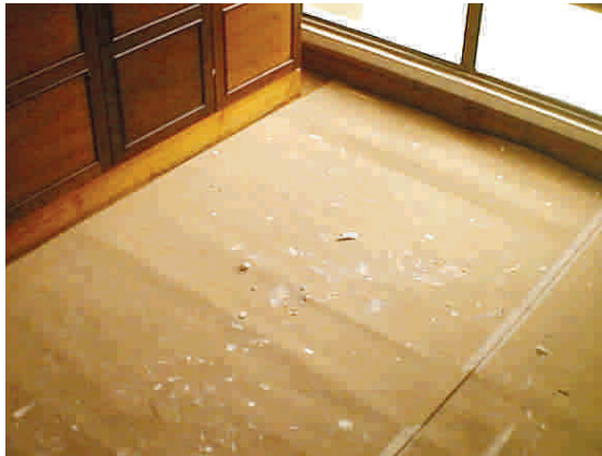
Protection of timber flooring with cardboards
