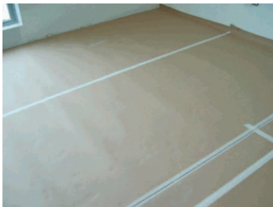
Protection of timber flooring with corrugated papers
