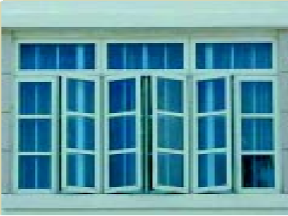
Window replaced or changed from sliding window to casement window
