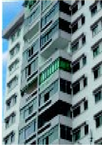
Residential building with some enclosed balconies
