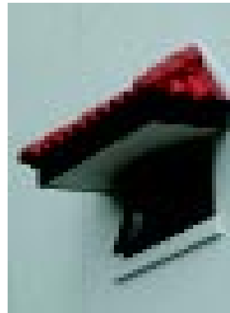
Windowhood with clay tile finish
