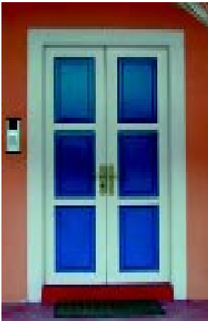
Door replaced from metal door to wooden door
