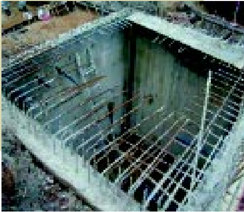
Vault (under construction)
