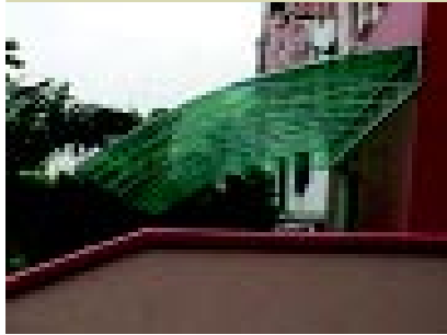
Cantilevered roof of lightweight material
