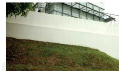
After repair: Reconstructed earth retaining wall
