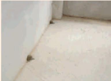
2.3. Apply a bonding agent (e.g. slurry coat) as per manufacturer's instructions.
