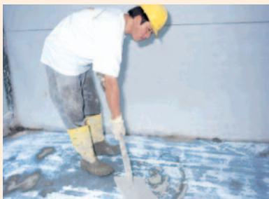
2.4. Tamp down the screed to remove any void and finish with trowel float and ensure no undulations.
