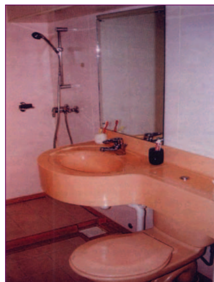
Figure 2.1: Interior of a prefabricated bathroom
