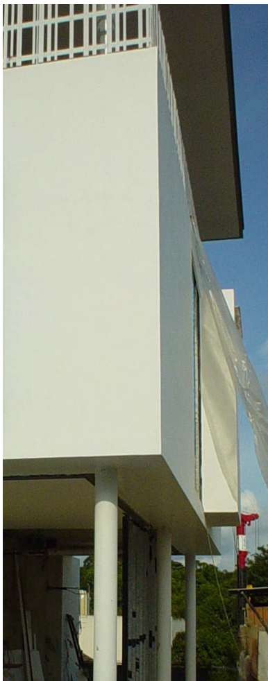
Figure 5.6 Semi-detached houses using flat plate with steel column (near completion) Designed by: IP:LI Architects
