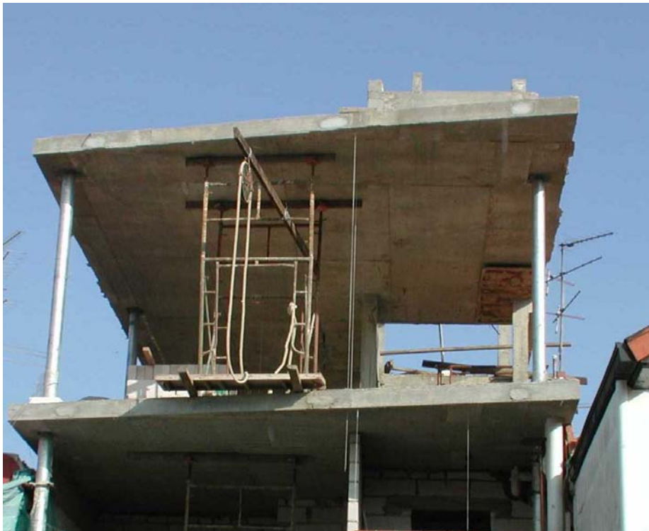
Flat plate system with circular steel column
