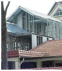
**Strong but Lightweight:** Steel has one of the highest strength-to-weight ratios of any construction material. This results in savings in the foundation required and the lightness also makes for easier on-site handling.
