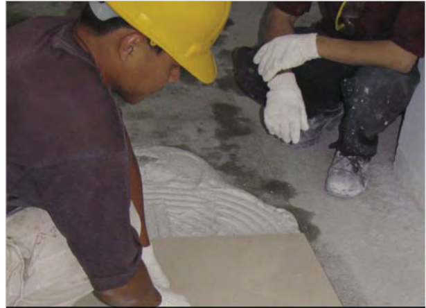
Fig. 1.6 - Screed-less flooring installation: Better productivity and quality.
