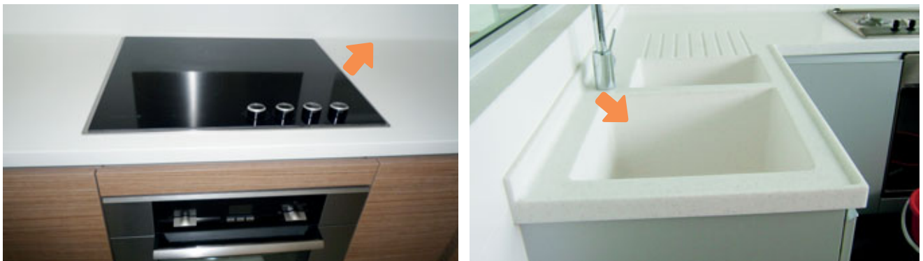
Fig. 2.6 – Sink and back-splash can be integrated in solid surface materials but not when using engineered quartz stone.
