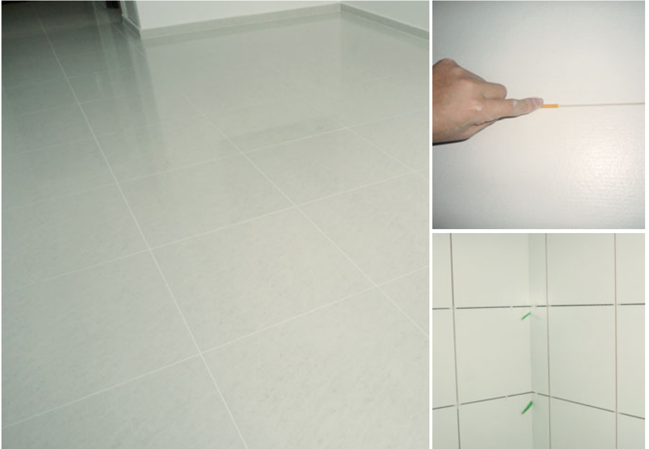
Fig. 3.7 – Good dimensional tiles aid better consistency in joints.
