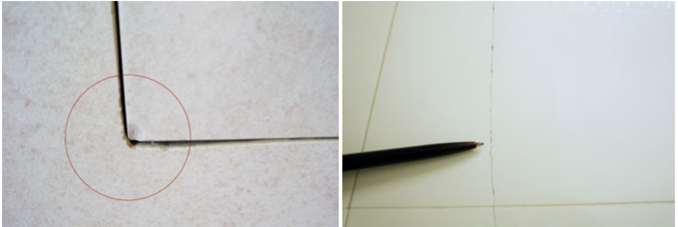
Fig. 3.11 – Tiles with low MOH rating are not suitable for heavy traffic areas.
