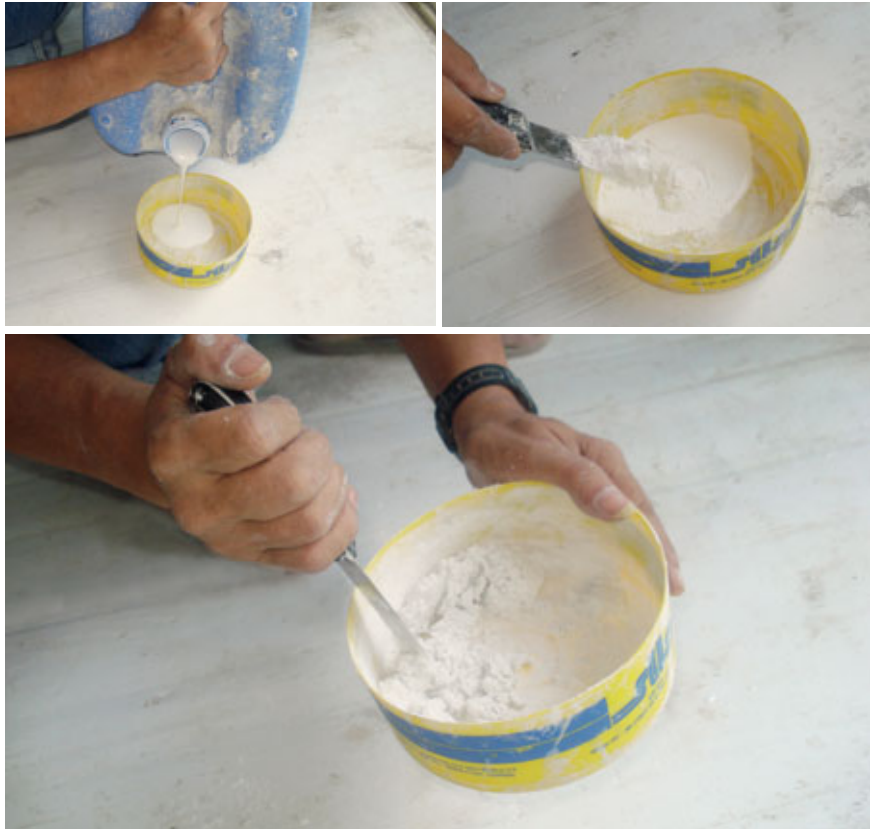
Fig. 6.1 – Adding liquid polymeric additives to cement grout enhances its performance.
