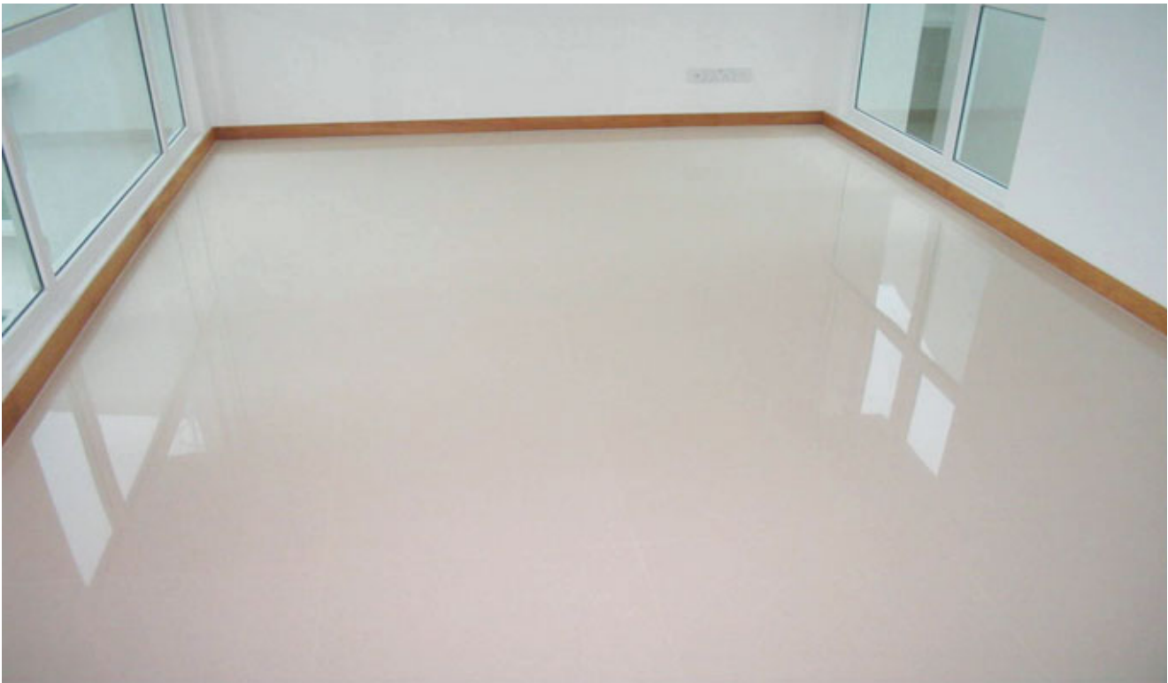
Fig. 6.7 – Better aesthetics and smoother joints on a marble floor using epoxy grout after polishing.
