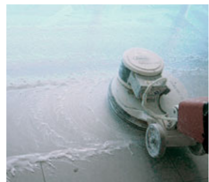
Fig. 6.3 – Wet polishing on a marble floor.
