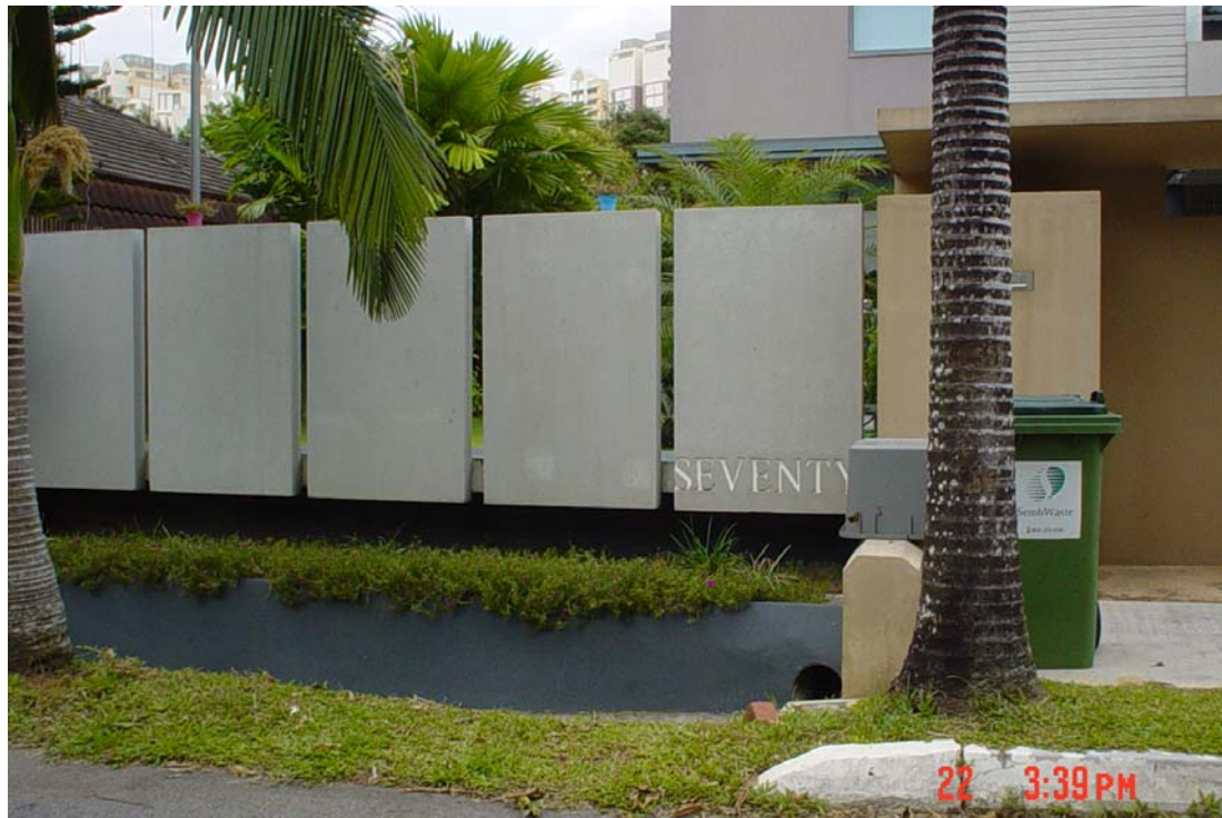
Figure 11.9 Completed view of the precast boundary panel walls
