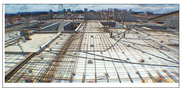
Figure 3.29 Option 1 - Services laid within the cast in-situ topping over the PC slab
